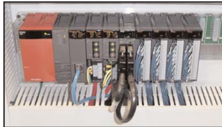
Q Series rack with 2 CC-Link Masters and other modules
