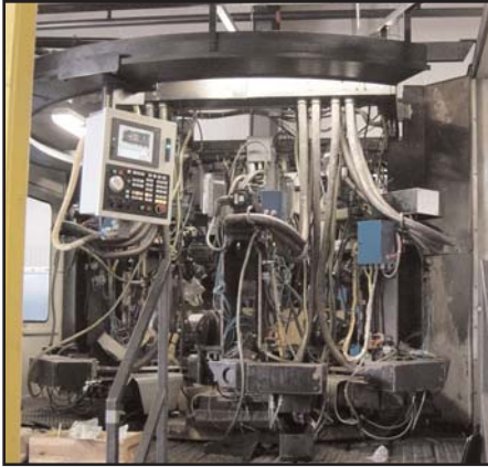
CNC Operator Interface on a moveable track
